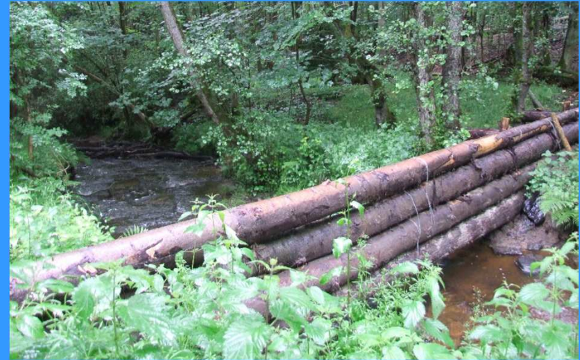
High level timber dams
